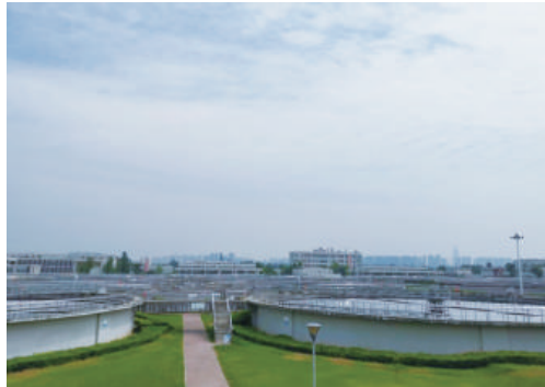
A sewage treatment plant of Chengdu Environment Investment Group Co., Ltd.
