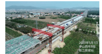
Bansantiliang Station, Section B, Zhongshan West Ring
