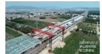
Bansantiliang Station, Section B, Zhongshan West Ring
