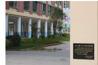
The IB Experimental Building in No.2 Experimental Elementary School in Zhenghe County built with the donation of IB
