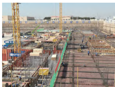
On-site construction of Xi'an Aerospace City Water Plant and Supporting Projects.
