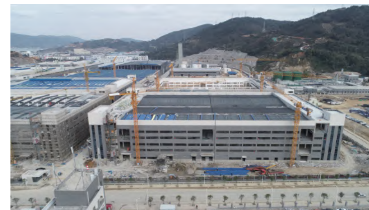
Industrial plant of Ningde Bangpu Circular Economy Technology Co., Ltd.
